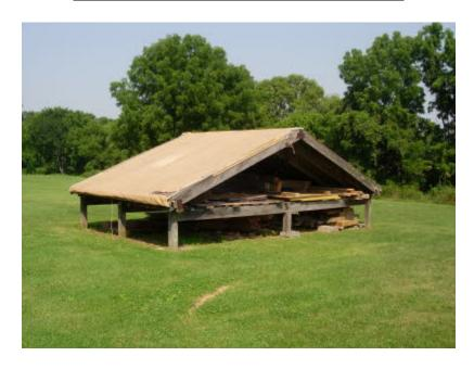
The roof ventilation simulator is constructed of lightweight truss and covered with 4x8 panels of decking materials.
